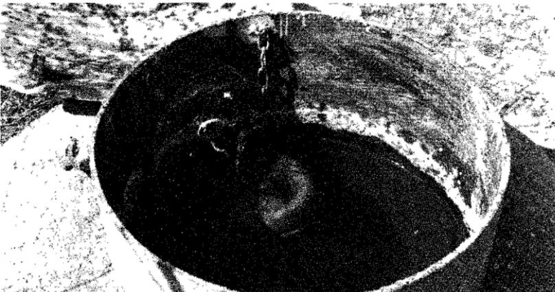
*Float-valve regulates water level in stock tank.*
